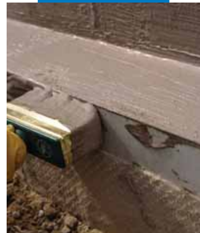
Waterproofing vertical walls with Mapeproof and Mapeproof Smart
