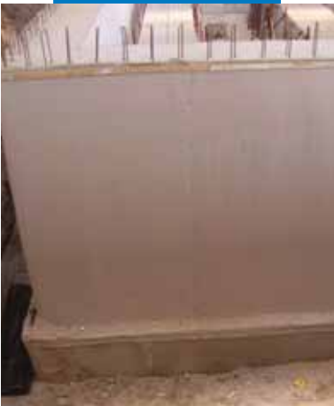
Waterproofing vertical surfaces after casting
