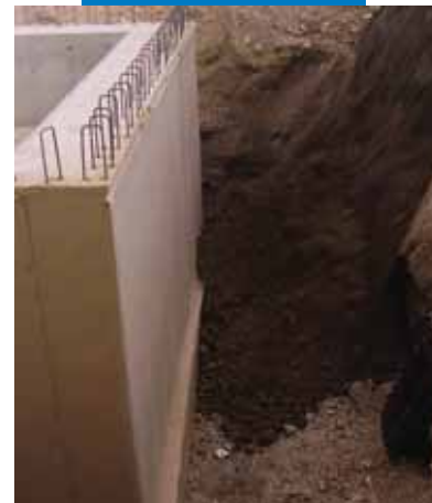
Filling in a trench
