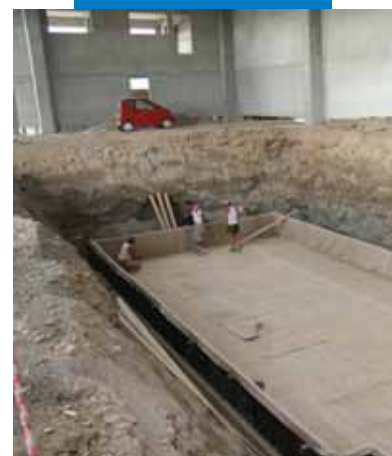
Waterproofing a horizontal surface with Mapeproof
