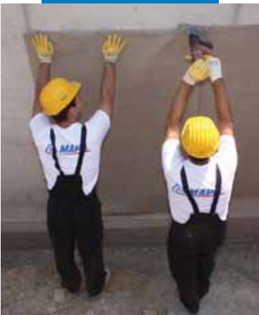
Fastening Mapeproof on a vertical surface using Mapeproof CD washers
