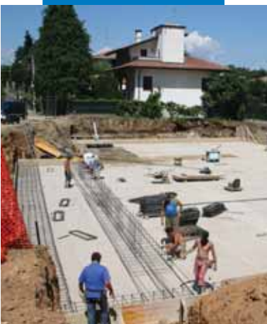
Waterproofing the foundations of a house
